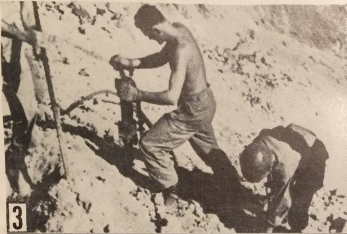
PINCHBARS, SHOVELS AND JACK-HAMMERS BLAST A LIP IN THE CLIFFSIDE RUBBLE.
