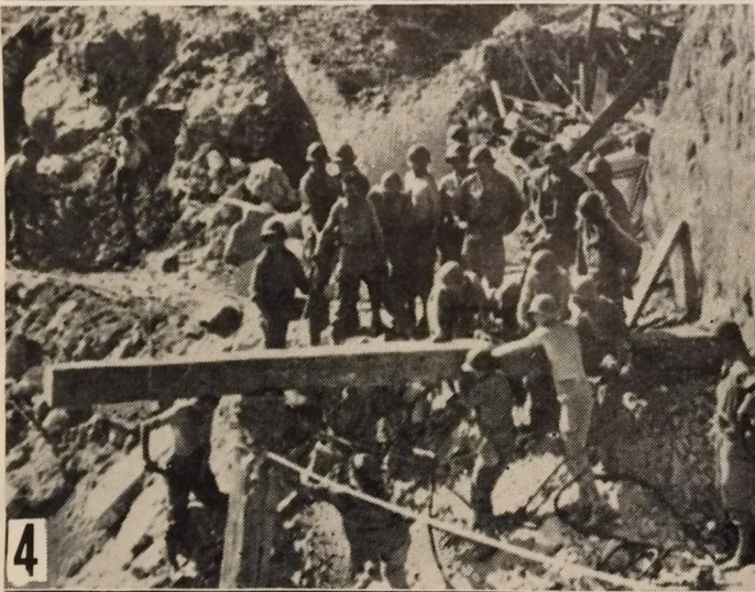
TIMBERS SWING INTO PLACE ON THE PERILOUS SLOPE. ROPES KEEP THEM STEADY.
