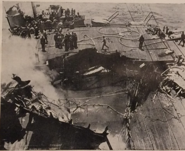
Gaping hole made by 500-lb. bomb.
